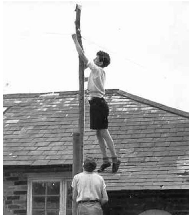
Stringing telephone cables to the Bunce Court cottage
